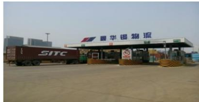
TIANJIN NEW HUAXI LOGISTICS
