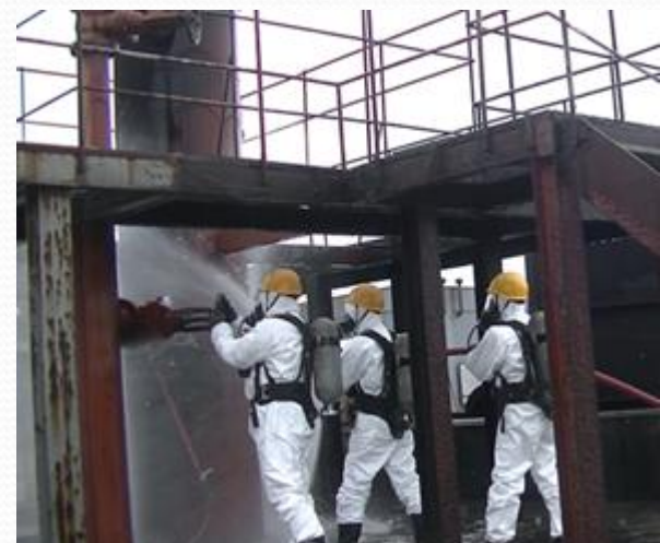
Dilution by water spray for HNS gas concentration
